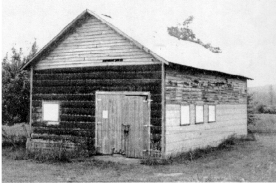
Burfiend butchering shed (ca. 1920) – exterior, looking to southeast
