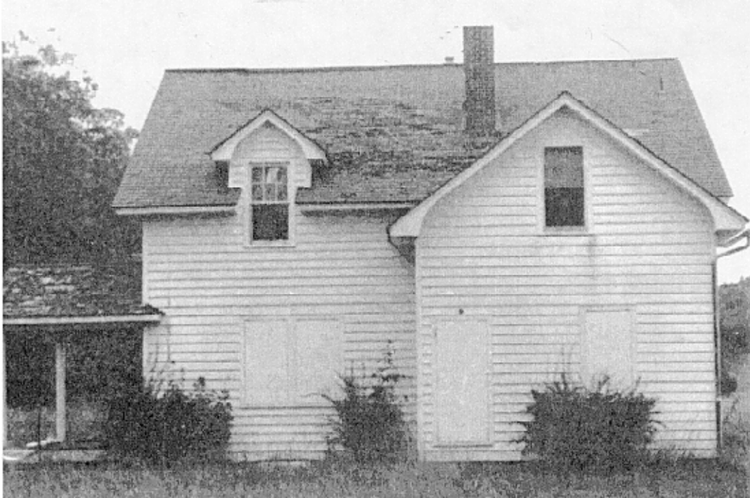
Figure 40. Burfiend house #2, 1993 (view to north).
