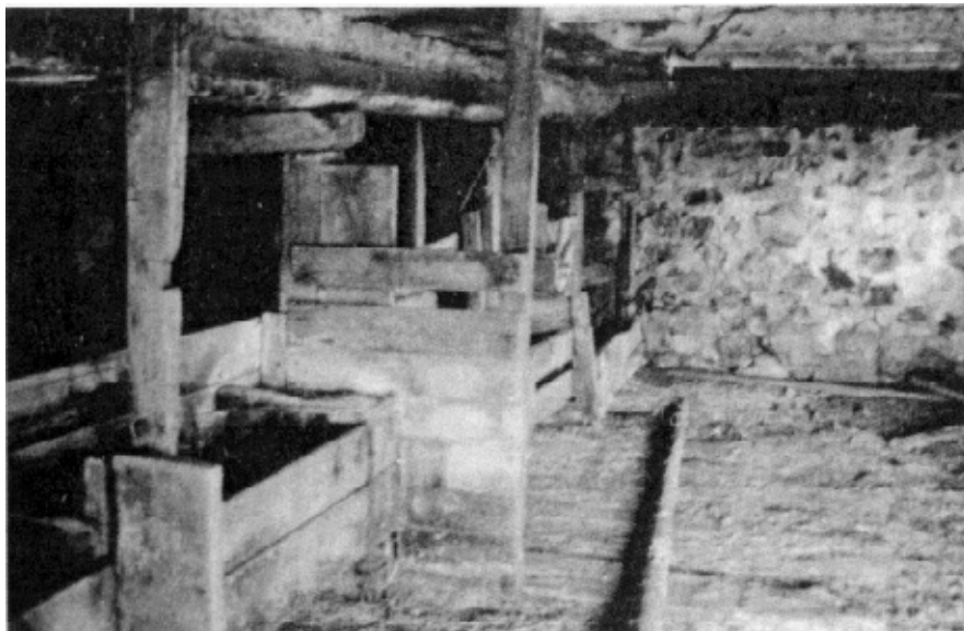
Howard Olsen barn – interior of basement, showing cow stalls
