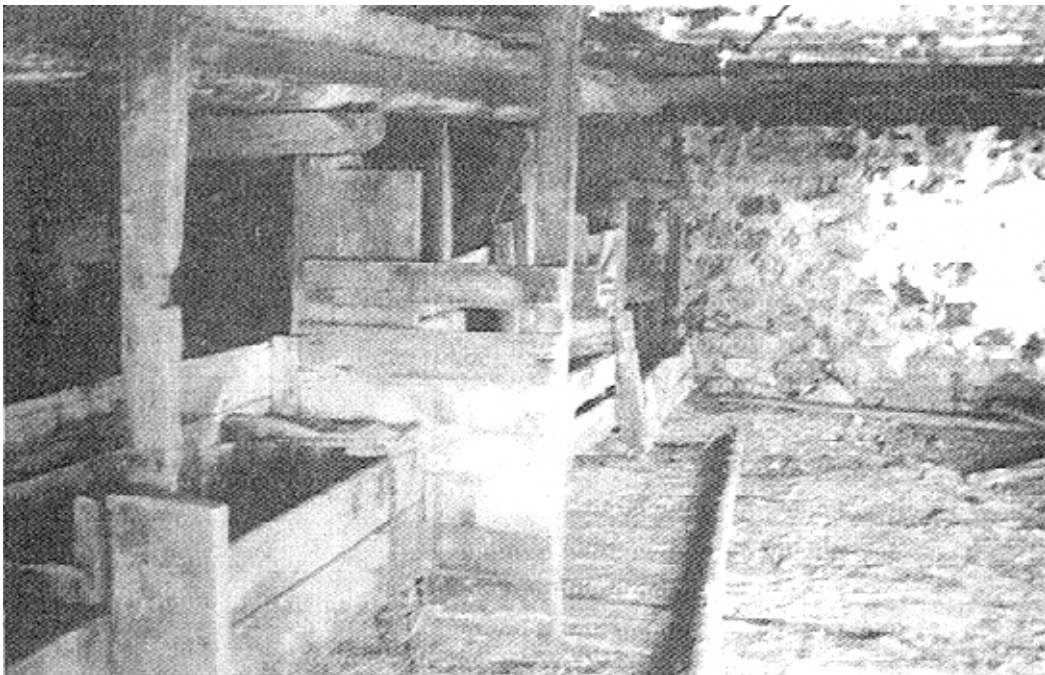
Figure 83. Interior of ground level floor for dairy barn on Howard and Bertha Olsen farm, 1993
