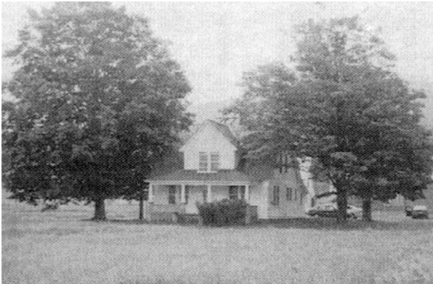
Dechow/Klett House, looking to south.
