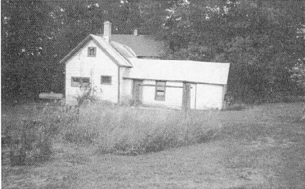
Figure 80. House on Howard and Bertha Olsen farm, 1993 (view to southwest).
