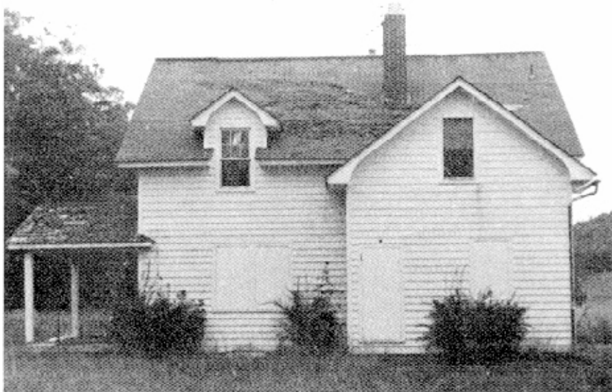
House #2 (ca. 1920) -- looking to north
