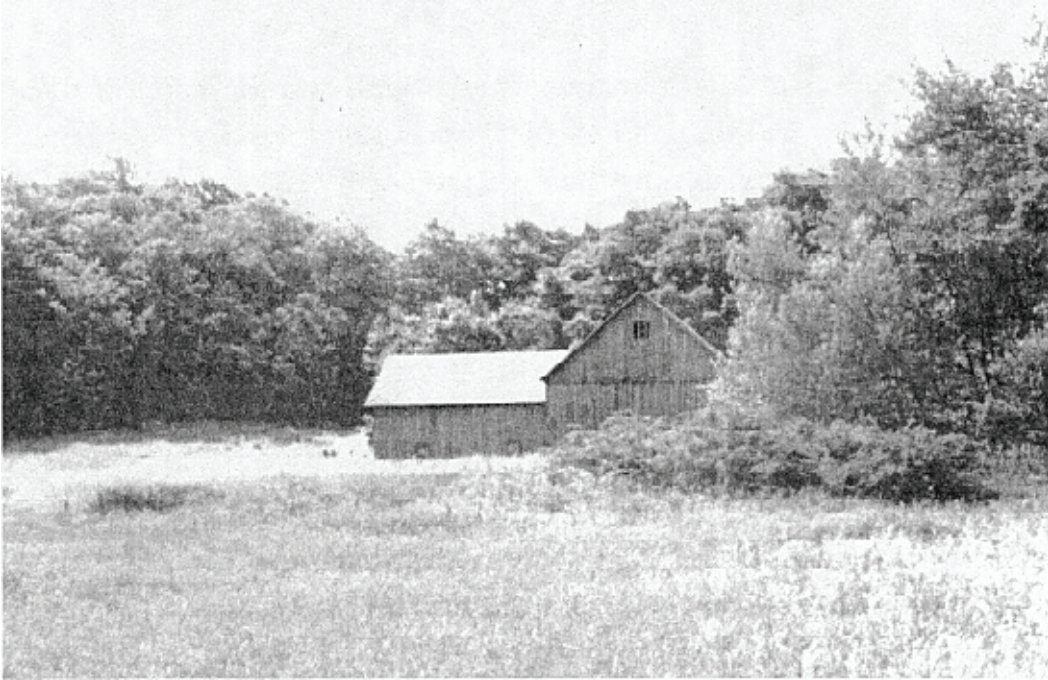
Figure 20. Miller barn, 1993 (view to south).
