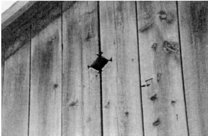
Schnor barn – gable end cutout
