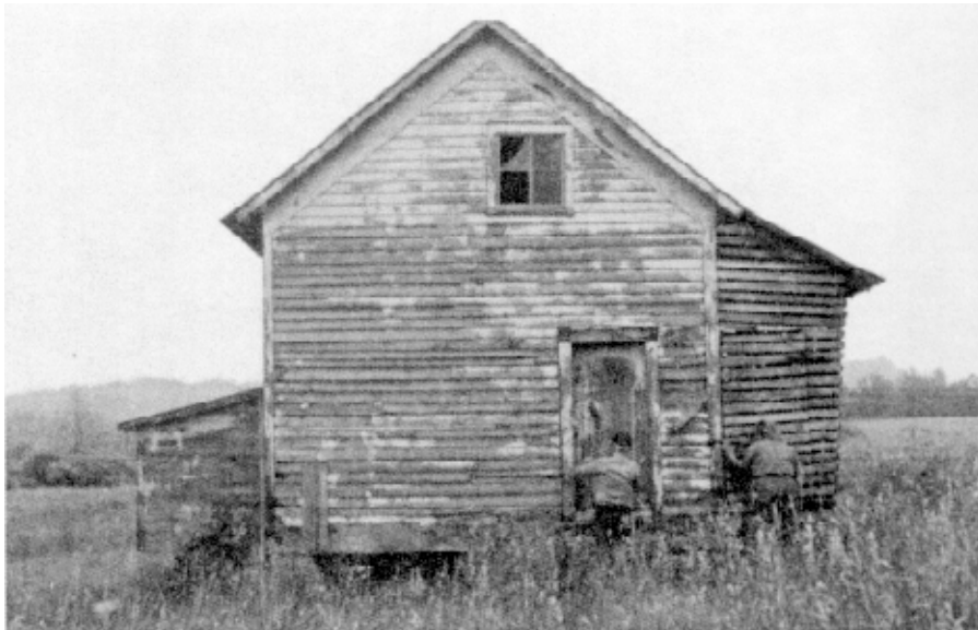
Burfiend farm – attached granary and
