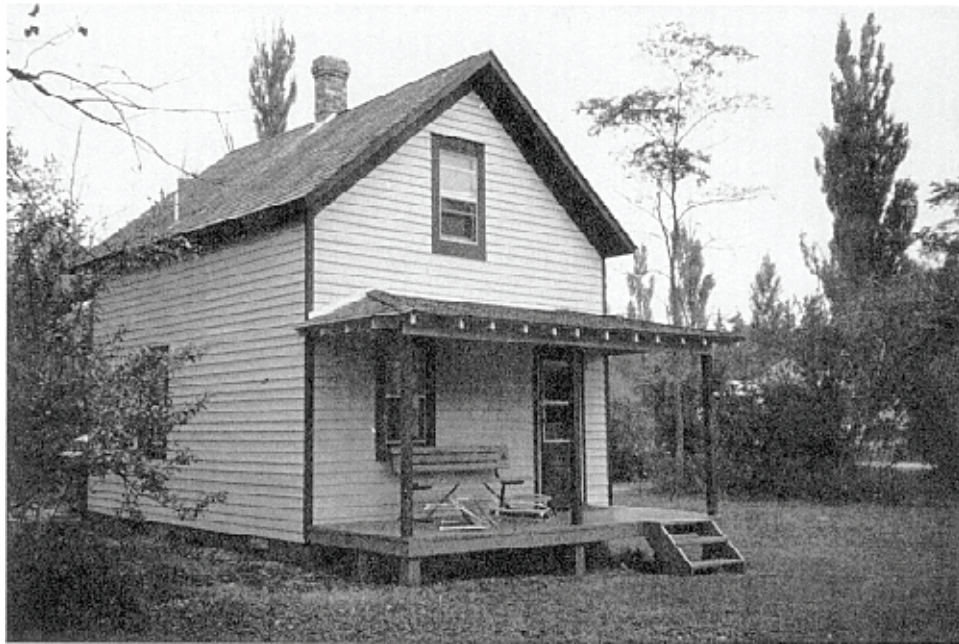
Figure 20. SMI Village Leinbach House, built ca. 1930 (1994)
