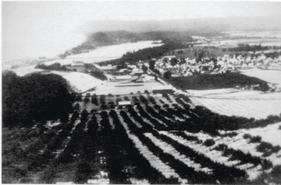
Figure 30. View of Empire village from from Orchard Hill looking north, early twentieth century.
